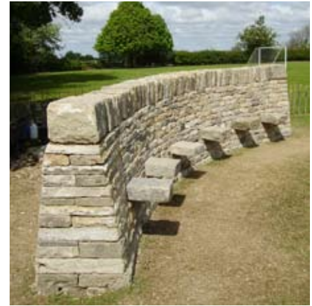
Traditional, dry wall of reclaimed stone, built at a school. Students put a time capsule in the wall. Wall & photo by Tracey Blackwell, Yorkshire.
