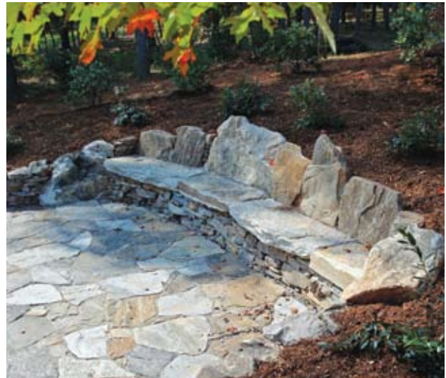
Green construction was a project focus when Biltmore Farms and Handmade in America started the Handmade House in the Ramble. This retaining wall, patio and bench are all dry laid using only locally sourced stone. My work with The Unturned Stone.
