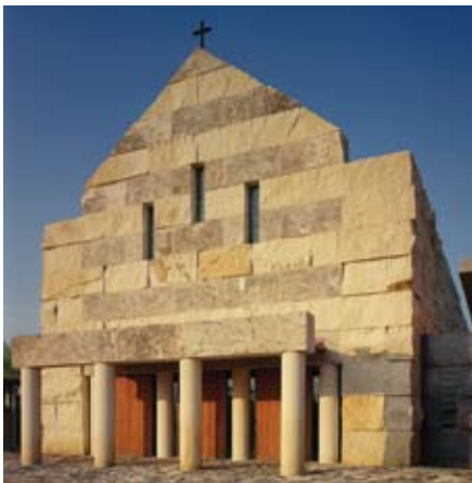
Our Lady of Dallas, Cistercian Abbey. Modern, load-bearing structural limestone. Photo by James F. Wilson, courtesy of Stonexus Magazine
