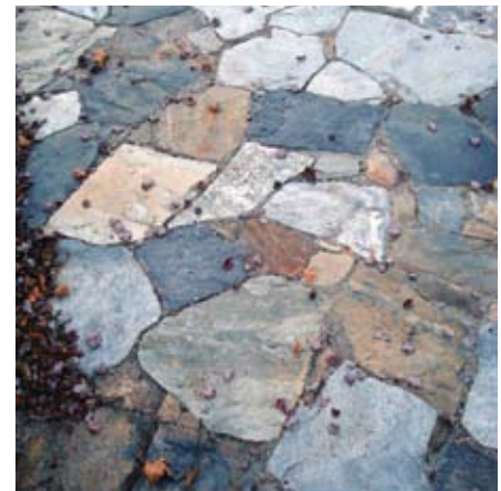
Flagstone laid on pea gravel bed drains water and will last longer than a mortared surface. Local stone. My work with Unturned Stone.
