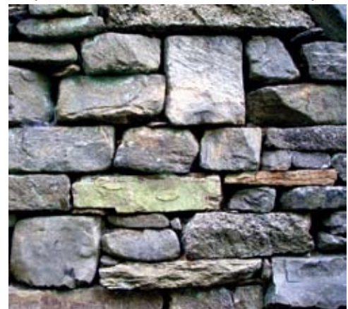
Detail of drystone retaining wall of local fieldstone
